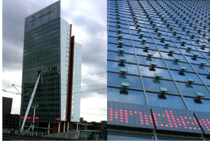
Figure 4.17: Left: KPN building by Renzo Piano. Right: closeup of display system, with additional standard ticker-style display.
